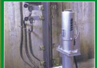
SPRING / HYDRAULIC BUFFER
